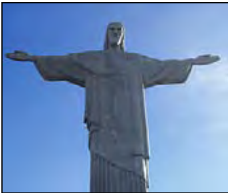
The outer layers of the Christ the Redeemer in Rio de Janeiro are made of soapstone.
